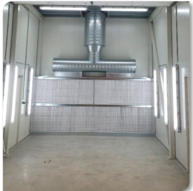
Above: Extraction in the rear wall.
