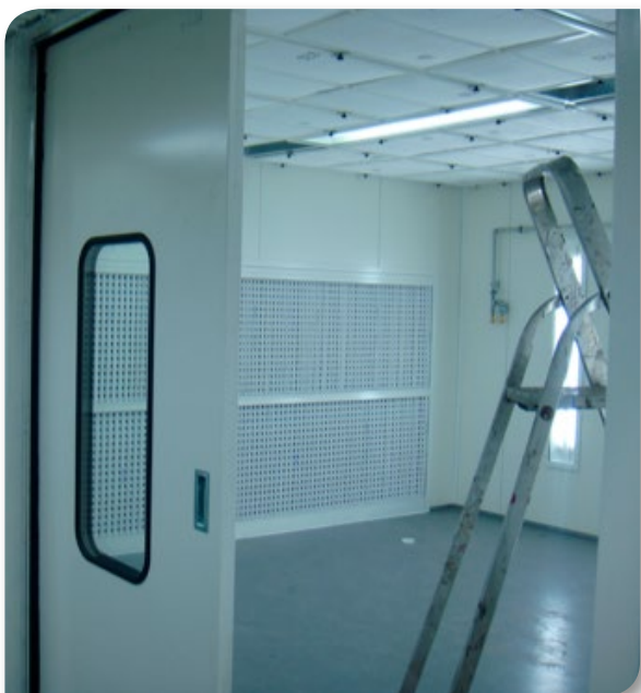
Above: Halden Fengsel, Norway. Extraction in the rear wall, injection in the ceiling.
