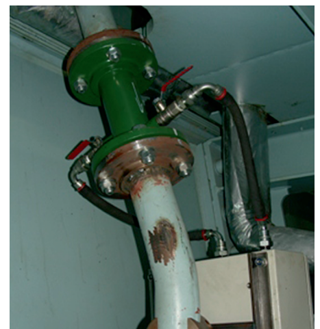
Baffle Section installed
